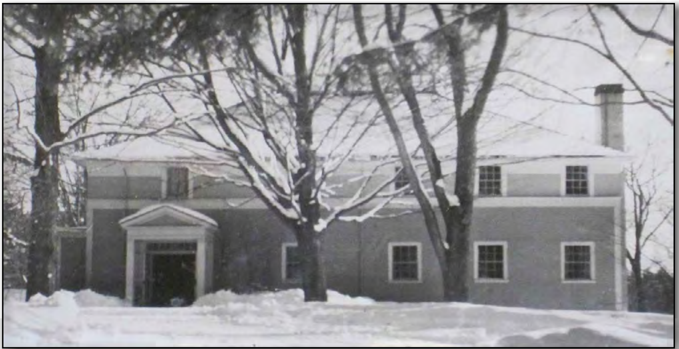
Thayer Hall 's Upper Entrance to Dining Hall and Rooms
