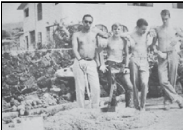
Building Wall In Mexico, 2nd Summer Outward Thrust Trip - 1963
